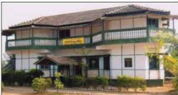
Kindergarten & Primary School at Diksal
